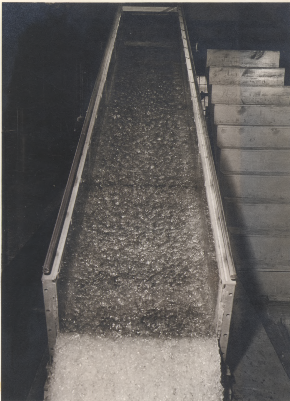
Figure 18 (a). Water Surface, Screen Boundary, 20° Slope, 1.22 csf/ft.
